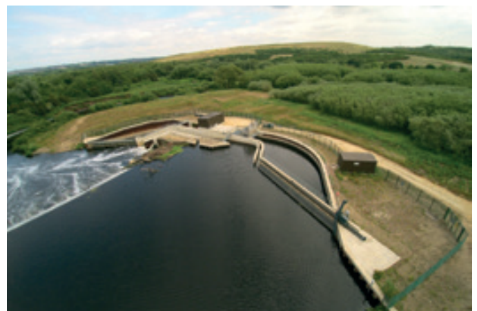
Thrybergh Hydropower plant
